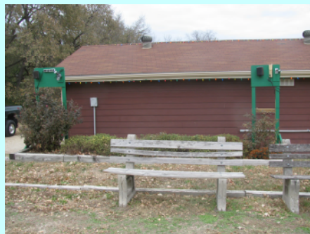
Green Supports Installed - Supports Netters Lights & Stereo Speakers
