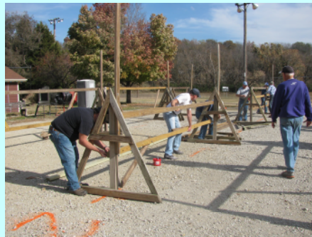
Assembling the 16' Stringers to the A-Frames
