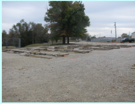
A-Frames and 16' Stringers laid out for assembly on Nov 5
