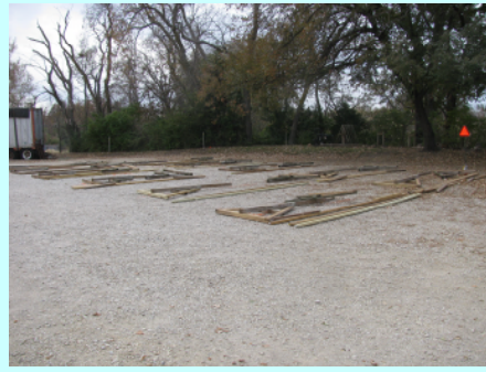
A-Frames and 16' Stringers laid out for assembly on Nov 5
